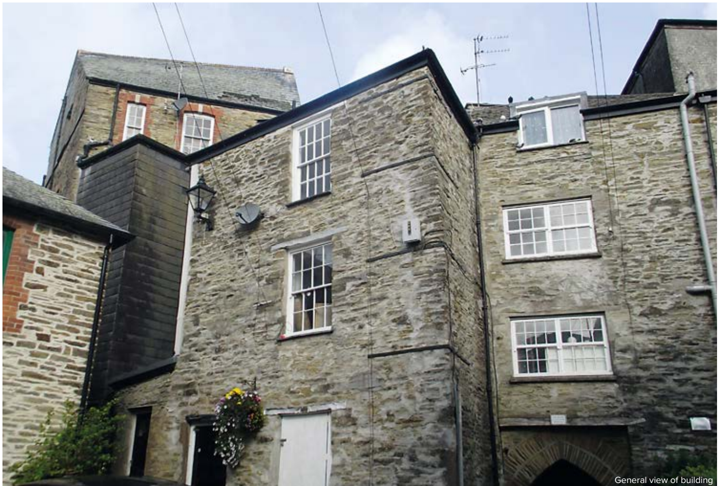
General view of building
